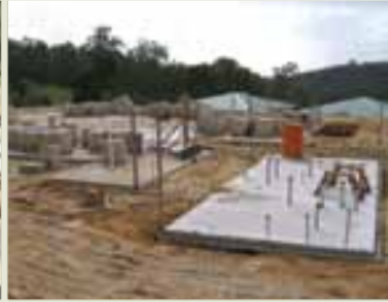
Dining complex foundations, 14 Sept. 2008
