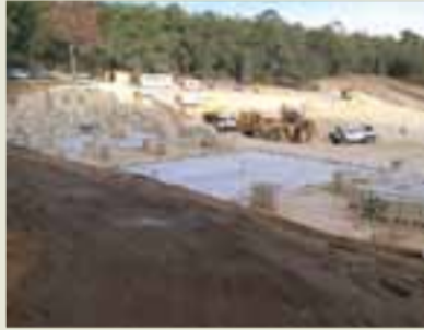
Cottage foundations, 29 Mar. 2008
