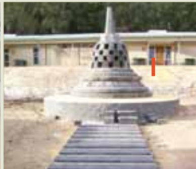
Stupa construction, 29 Mar. 2009
