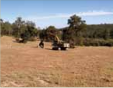
Clearing the ground, 16 Nov. 2007
