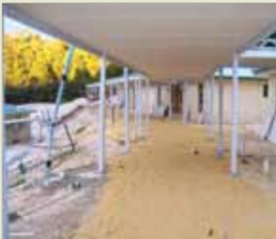
Walkway to the cottages, 29 Jan. 2009
