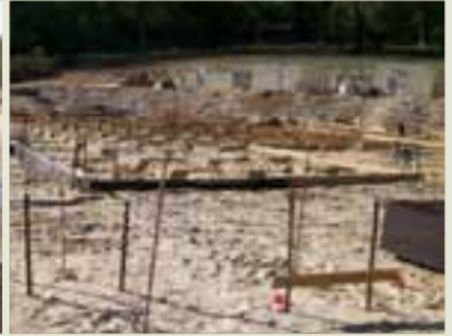
Meditation hall formwork, 2 May 2008
