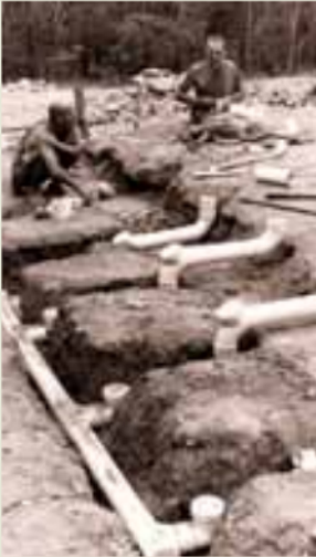
Ajahns Brahm and Jagaro doing pipe work for ablation block, 1984
