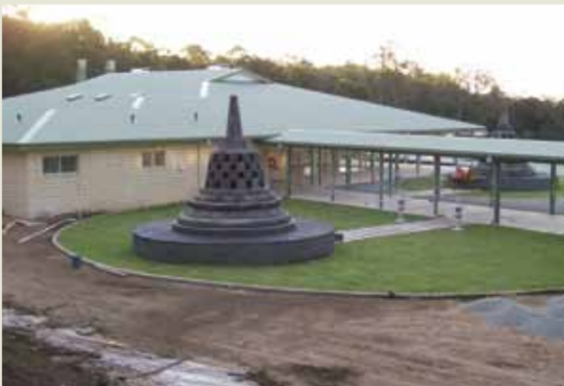
Lawns completed, 7 Apr. 2009
