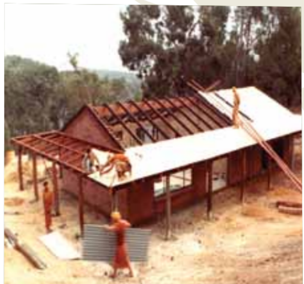
Building the dining hall of the monastery, 1985
