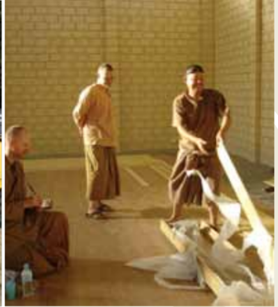
Monks working on the floor of the main hall into the early hours to complete it on time
